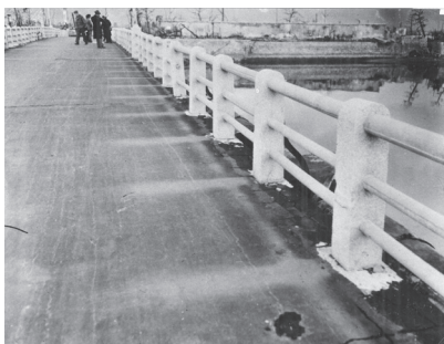
"Shadow of Railing (890m from the hypocenter Heat rays scorched and blackened the asphalt, but it remained white where the bridge railing blocked the rays.)"
